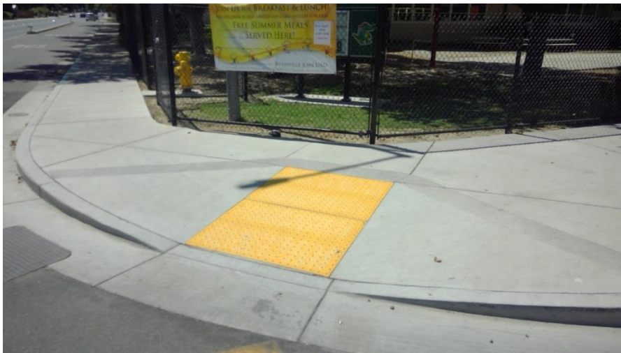
Figure 4: Example of curb ramp compliant with ADA standards (Data entry #38)
